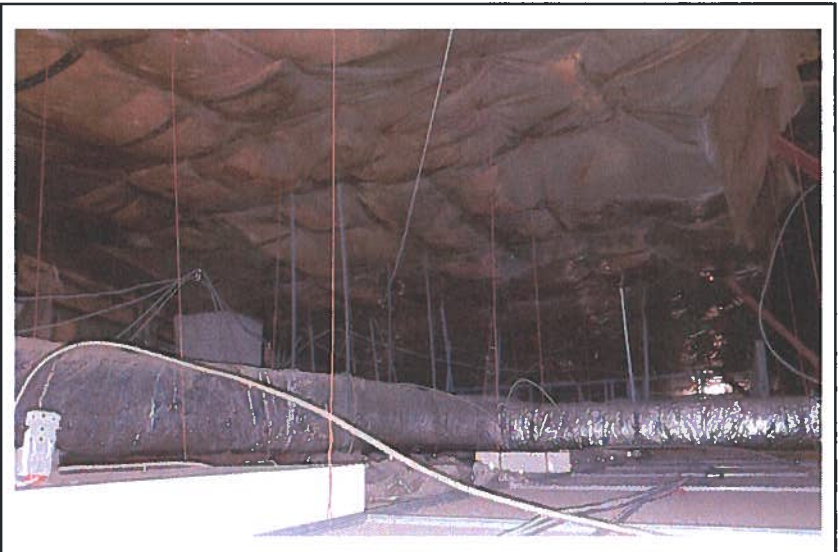
Photo 058 Insulation and Plastic Covering
