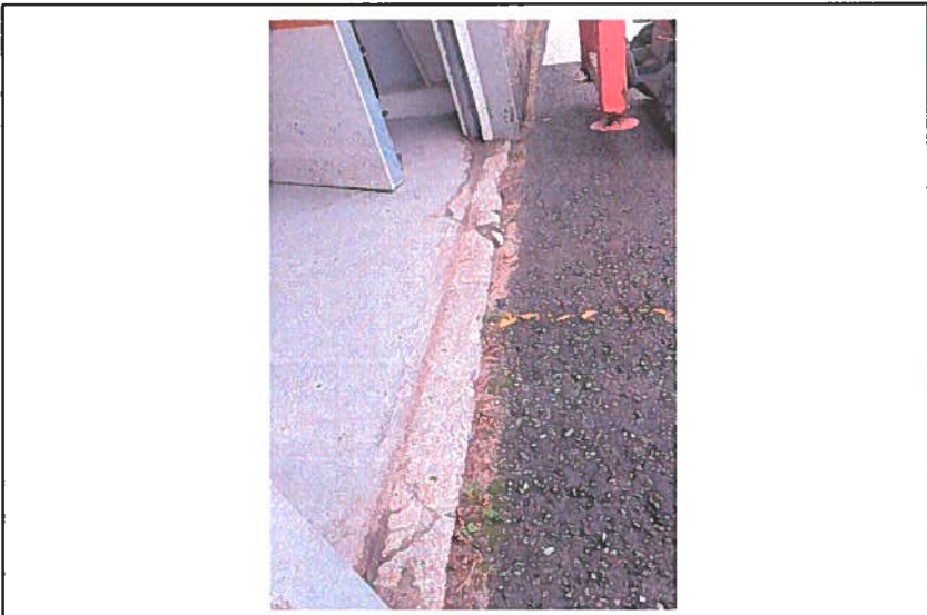
Photo 018 Apron Slab Under Garage Door
