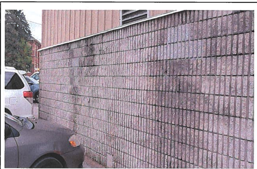
Photo 068 Architectural Precast Concrete Wall Panels
