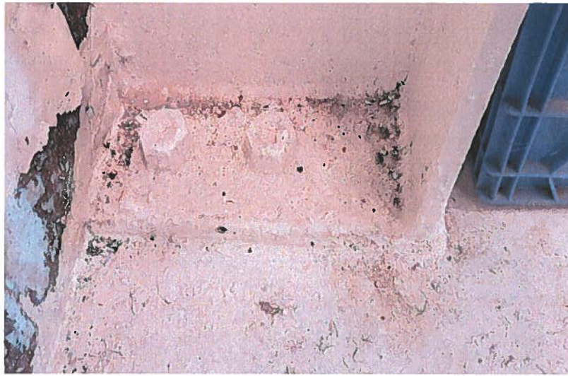
Photo 007 Pre-Eng Frame Base Connections
