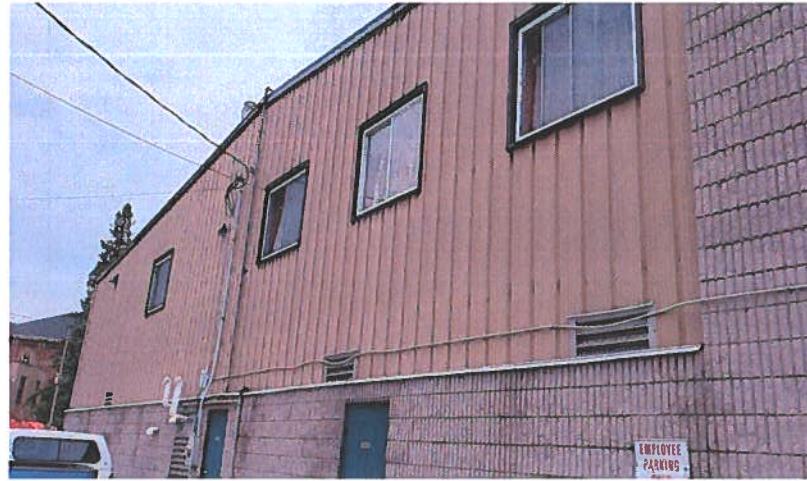
Photo 069 Metal Siding Along South Side
