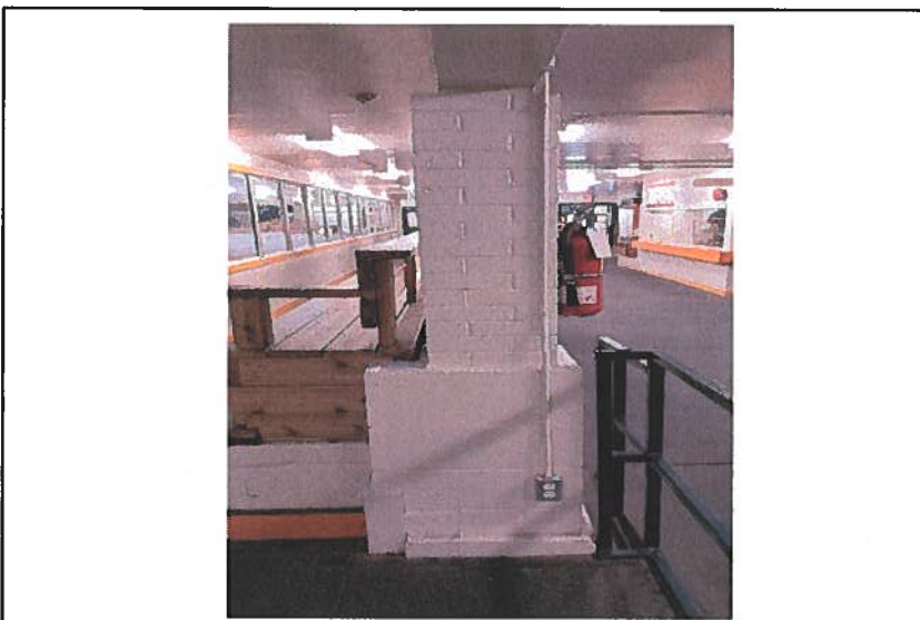
Photo 044 Columns in Lobby
