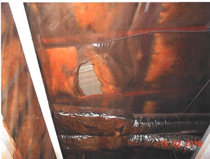
Roof Insulation Above Hall
