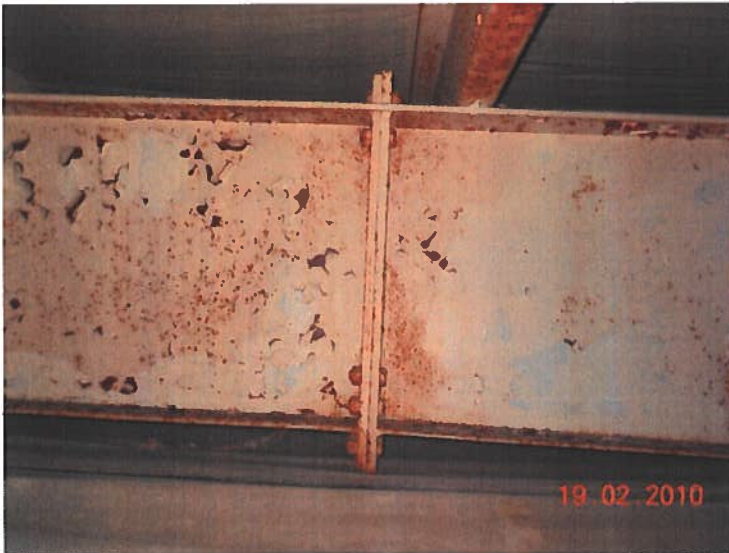
Steel Roof Framing Above Low E Ceiling
