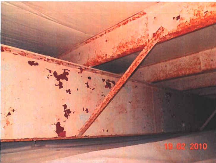
Steel Roof Framing Above Low E Ceiling
