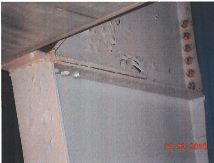
Steel Frame Eave Connection
