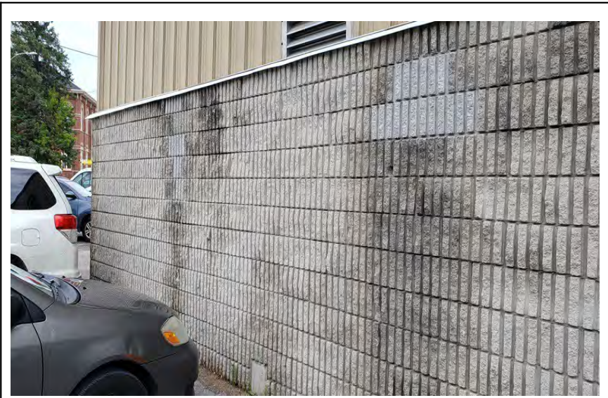
Photo 068 Architectural Precast Concrete Wall Panels
