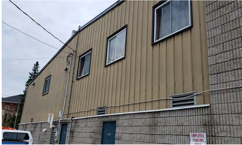
Photo 069 Metal Siding Along South Side
