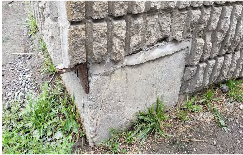
Photo 063 South-West Corner Foundation
