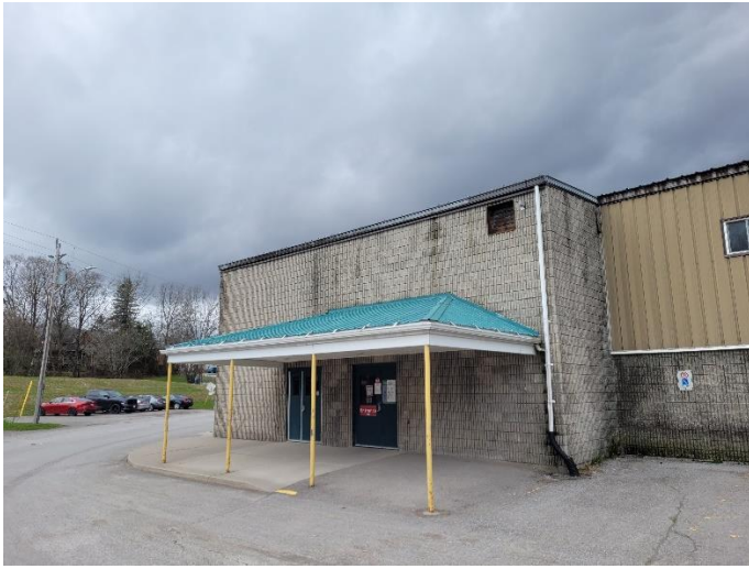
Photo 29 – Arena Entrance on East Elevation
