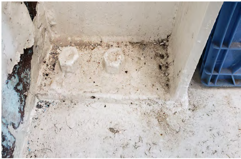
Photo 007 Pre-Eng Frame Base Connections
