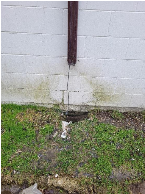
Photo 27 – Downspout at West Elevation
