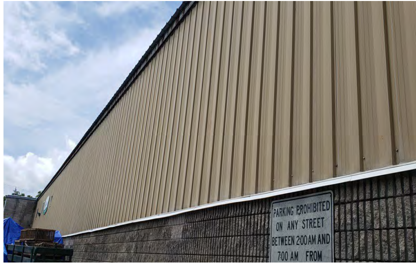
Photo 076 East Side Metal Cladding
