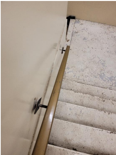
Photo 19 – Damaged Rail
