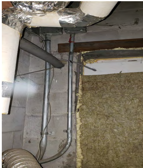
Photo 048 Localized Block Failure
