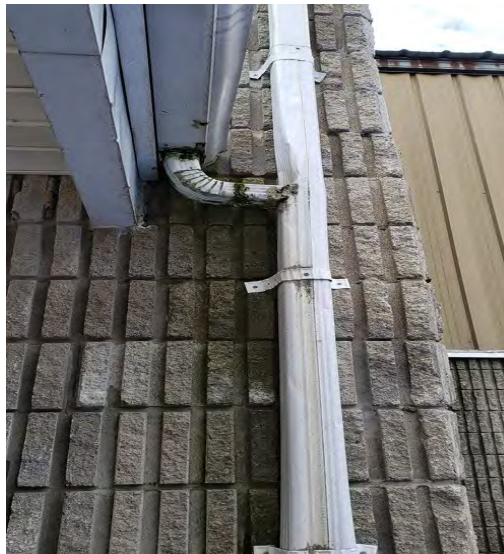
Photo 072 Damaged Eaves
