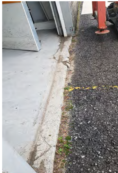
Photo 018 Apron Slab Under Garage Door
