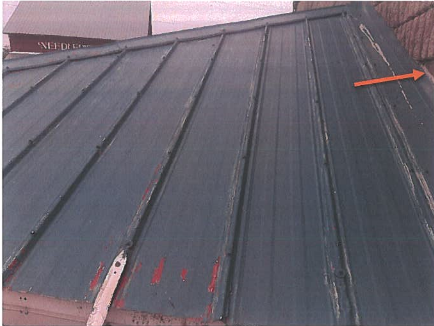
Photo 5 – Asbestos-containing white exterior caulking.
