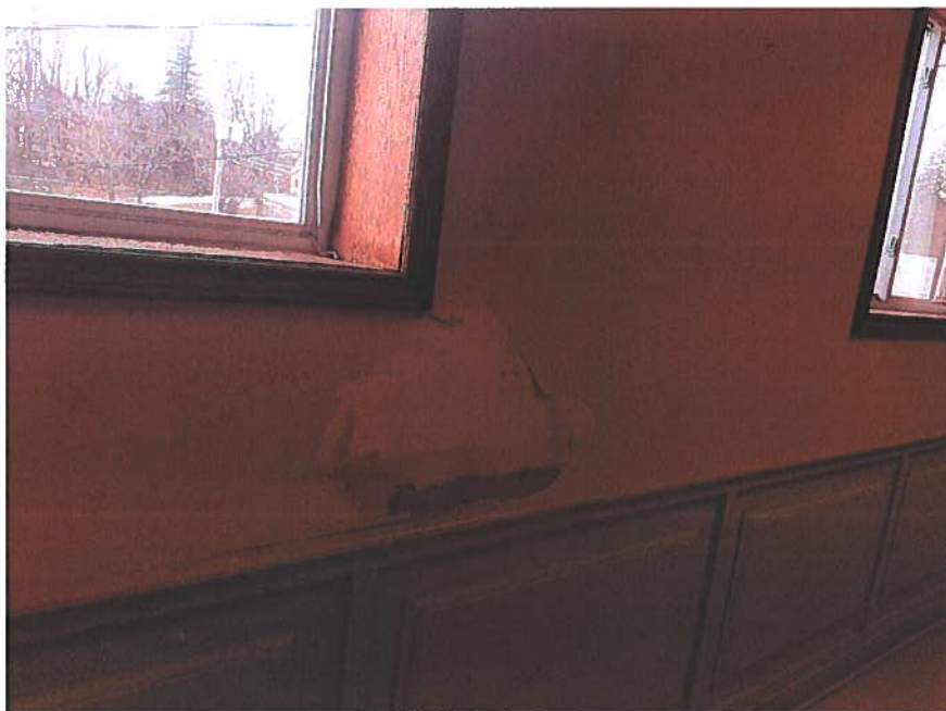
Photo 3 – Asbestos-containing drywall joint compound in poor condition.
