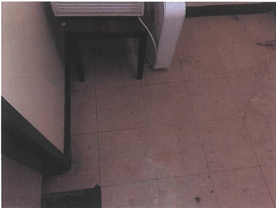
Photo 2 – Asbestos-containing vinyl floor tiles in the second floor.
